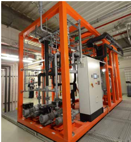
Congelo is an ammonia/water absorption chiller which generates cooling temperatures down to -30\text{ }^{\circ}\text{C}
